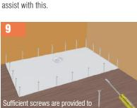
Use the longer screws provided to secure the ShowerDec® to the floor joists. Ensure ShowerDec® is secured along all 4 edges to eliminate any movement.
